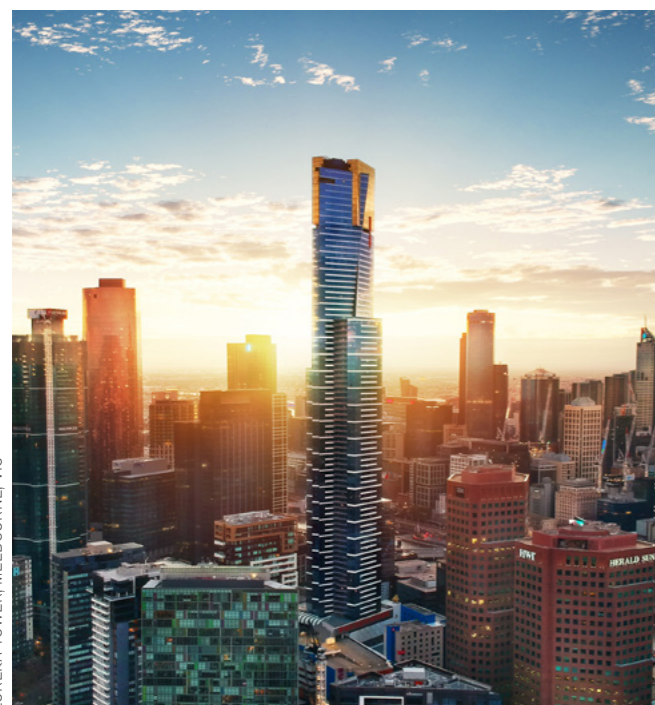
EUREKA TOWER, MELBOURNE, VIC
